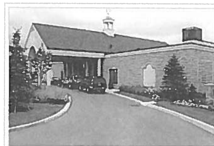
The Assumption Catholic Cemetery and Crematory in Mississauga, Canada, with chimney visible
