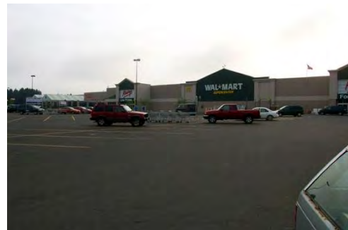
Typical Highway Commercial Use along State Highway 33
