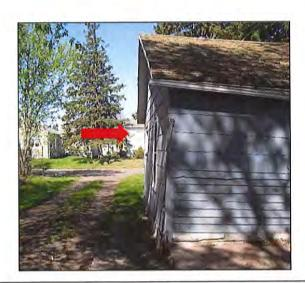
The first photo is the front of the home facing west. The home has settled on the exterior wall and the photo illustrates this settling. The second photo to the right, shows evidence of foundation failure indicated by walls out of plumb (out of proper alignment, not structurally sound, not level).
