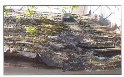
These photos show that there is extensive deterioration of the roof covering and underlayment materials. Furthermore, these photos show there has been no maintenance of the roof for a considerable amount of time, hence, the roof it well past its useful life and has led to deterioration internally of the home.
