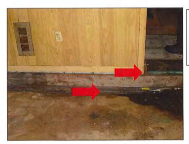
This photo illustrates the main level floor system failure. In this photo, the floor trim is where the floor is supposed to be, however the floor is not and it has actually sunk roughly 6 inches due to the foundation failure of the home.
