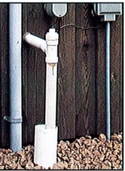
Sump pump discharge should go out through the wall into your yard or into a ditch.
