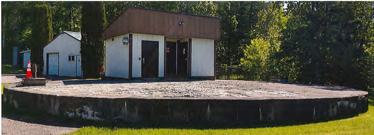
Spring Lake Pumphouse on Round Reservoir
