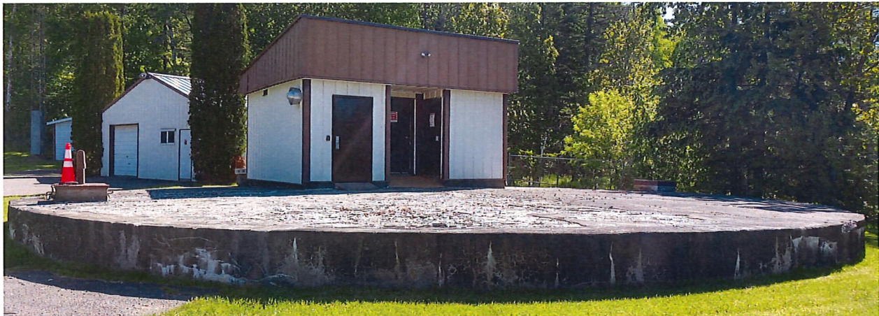
Spring Lake Pumphouse on Round Reservoir
