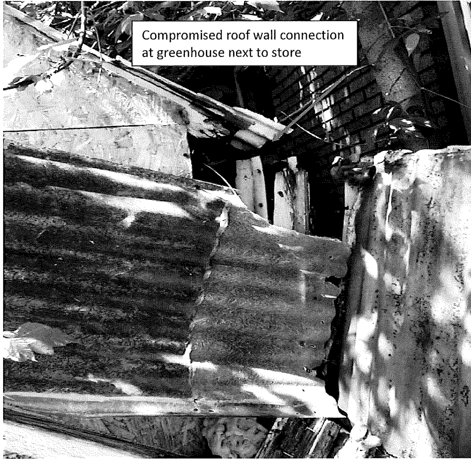
Collapsed Greenhouse
