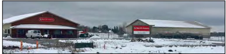
Best Oil purchased the former Cloquet Home Center and renovated the building into their office headquarters.
