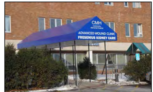
BELOW: Community Memorial Hospital constructed a wound clinic and kidney care, above is the new canopy entrance for that center.
