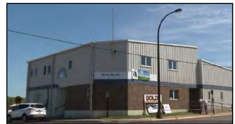
ABOVE: Friends of Animals purchased the former County Human Services Building on Avenue B and 10 th Street in Downtown Cloquet. Boldt Construction was the General Contractor and volunteered significant time as did many other businesses in the region to bring this project to reality. BELOW: new interior kennels.
