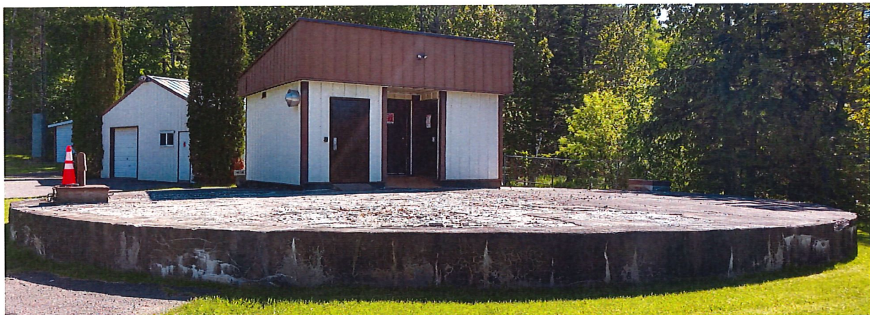
Spring Lake Pumphouse on Round Reservoir
