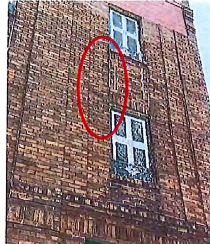
Sections of loose brick along the 10 th Street side of the building
