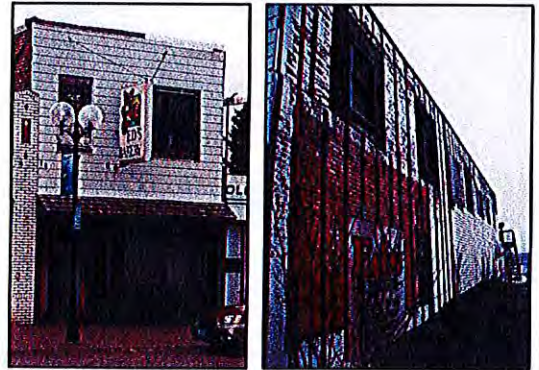
The Ed's Bakery building at 1013 Cloquet Avenue.
