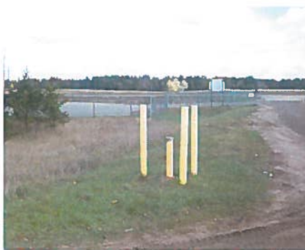
- Groundwater Monitoring Well
