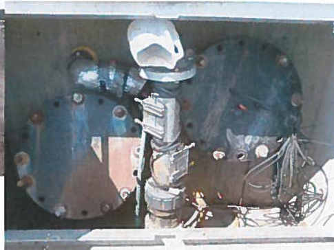
- Leachate Side-Slope Riser
