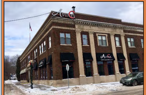
The Avenue C Restaurant recently opened in 2017 at 207 Avenue C, the historic First National Bank Building.
