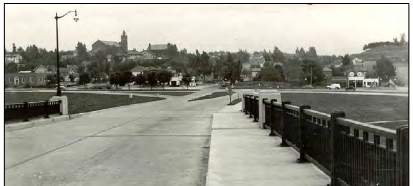
Highway 33 did not exist through Cloquet until the late 1960’s. This photo shows the intersection design and strong east-west roadway patterns with the south roadway simply being a residential street (now Highway 33 today).
