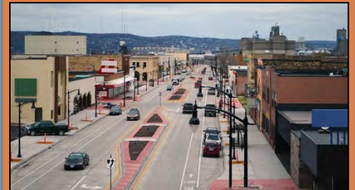
The recently completed Tower Avenue streetscaping project in Superior, WI.
