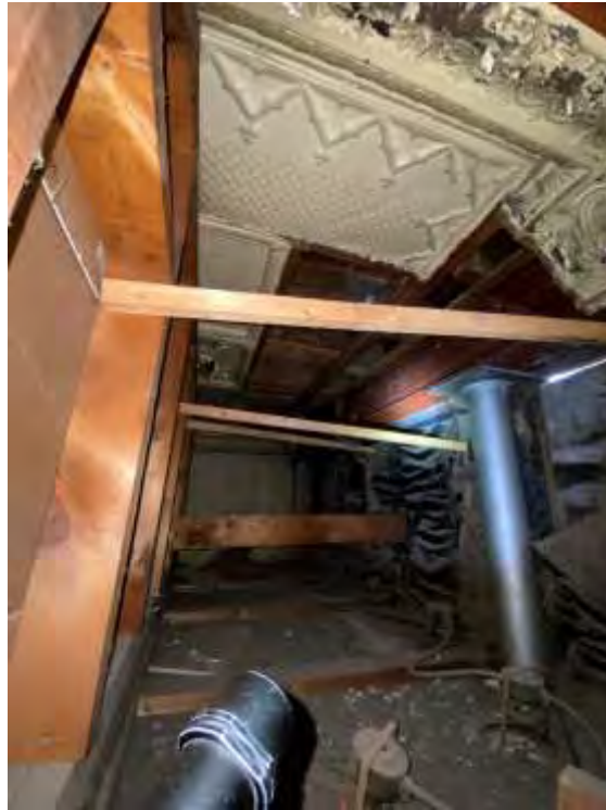
Photo 16: Steel Beam and Column
