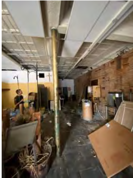
Photo 18: 2 nd Floor Soffits
