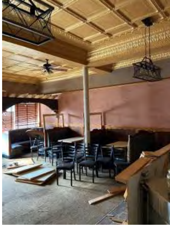
Photo 19: 2 nd Floor Soffits
