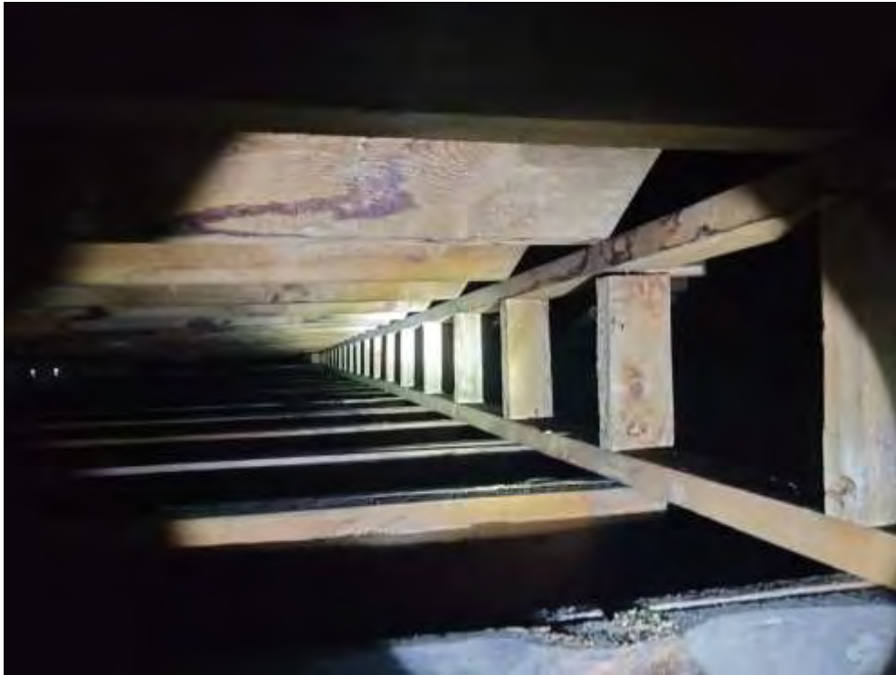
Photo 10: Interior Bearing of Roof Structure
