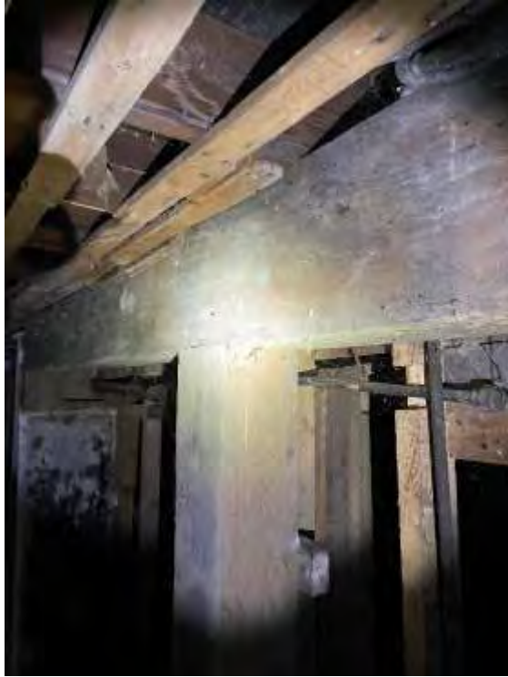
Photo 25: Wood Column to Girder
