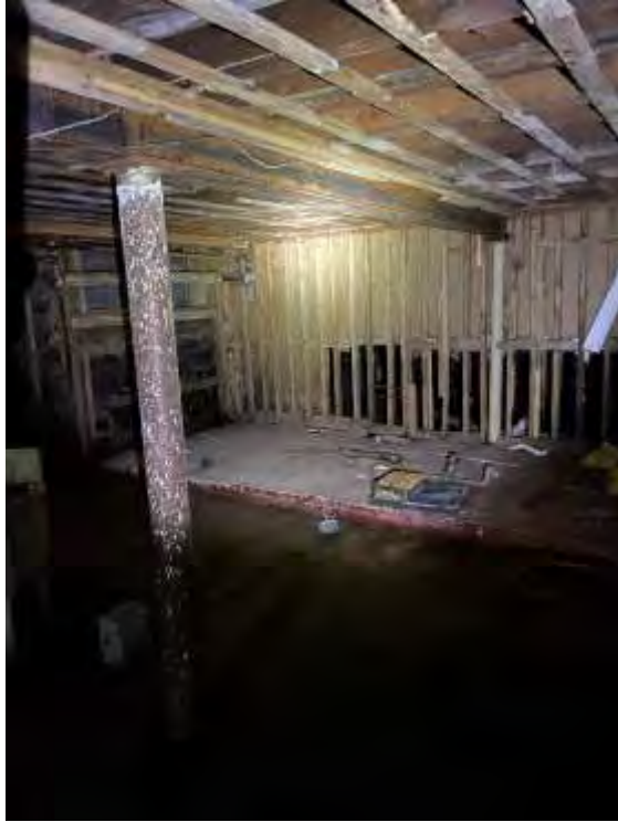
Photo 21: 1 st Floor Structure
