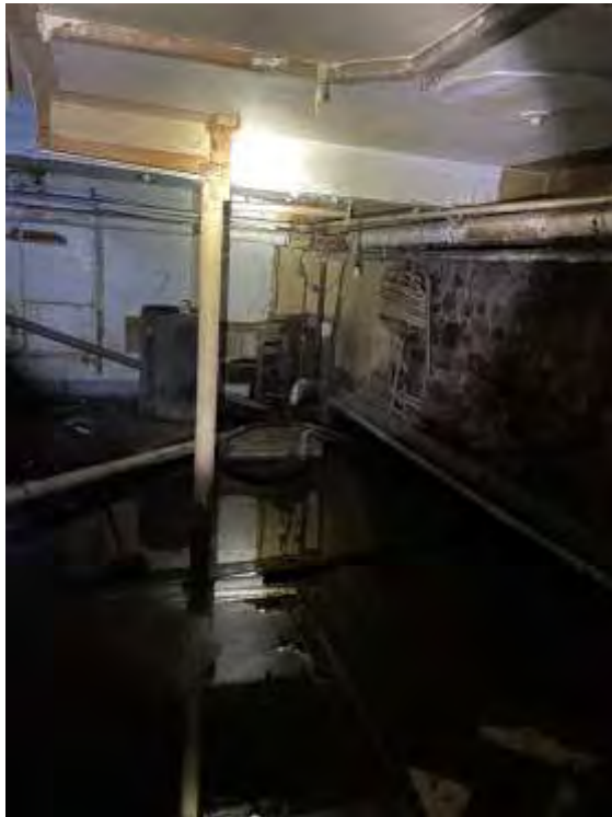
Photo 22: 1 st Floor Structure
