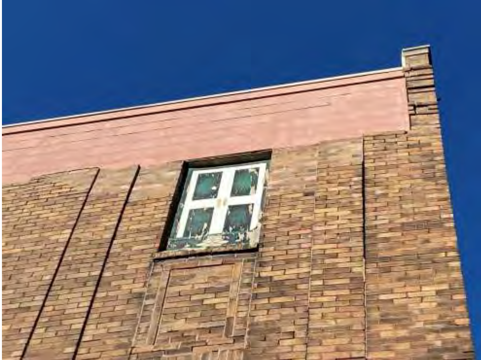
Photo 5: East Elevation Close-up
