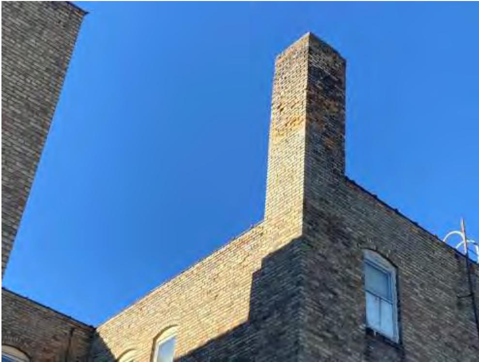
Photo 8: Chimney at North Elevation
