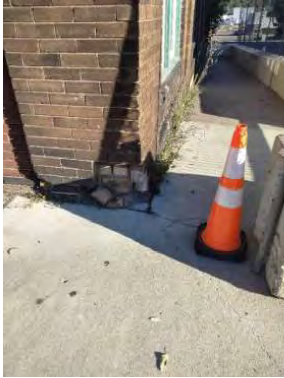
Photo 9: Missing Brick
