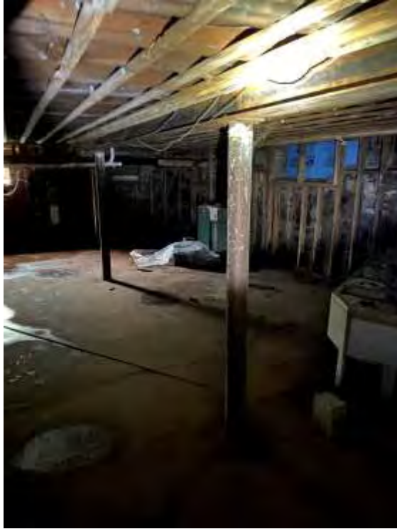
Photo 23: Steel Column and Girder
