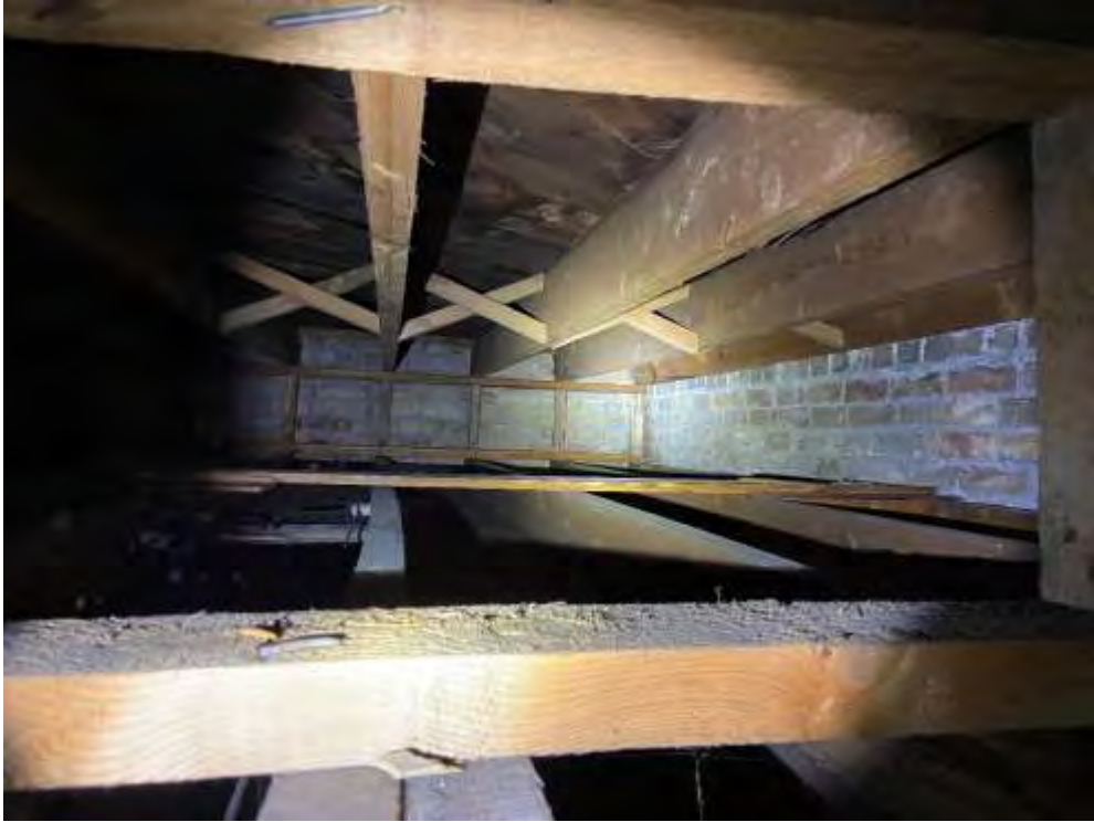
Photo 11: Exterior Bearing of Roof Structure
