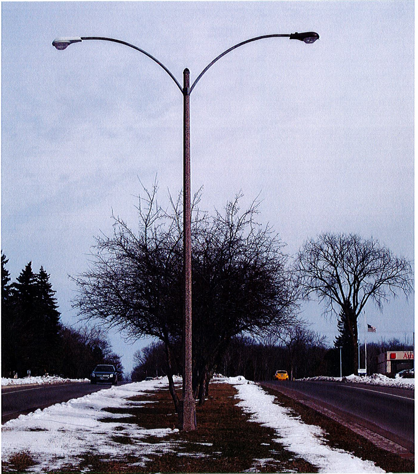
Concrete Poles – Approximate 20' Height – Approximate 10' Arms
